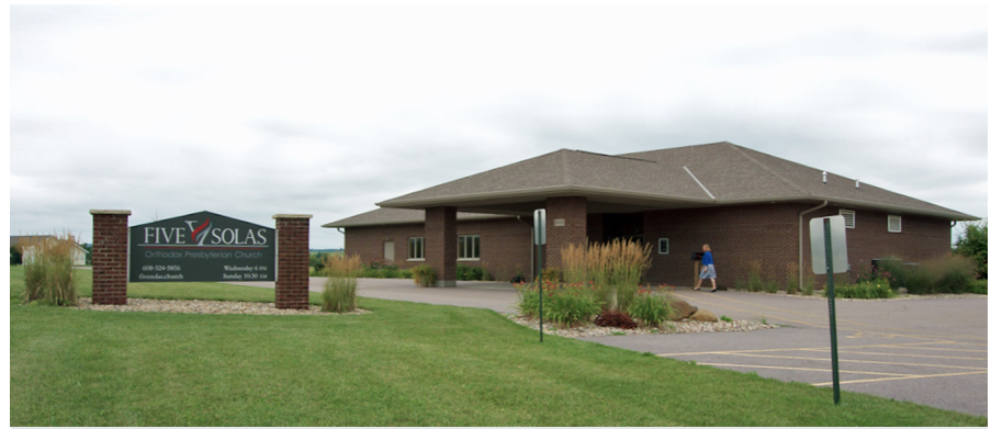
On September 20, Five Solas Reformed Church in Reedsburg, WI, which began as a mission work of the OPC, dedicated its new building with a special service
