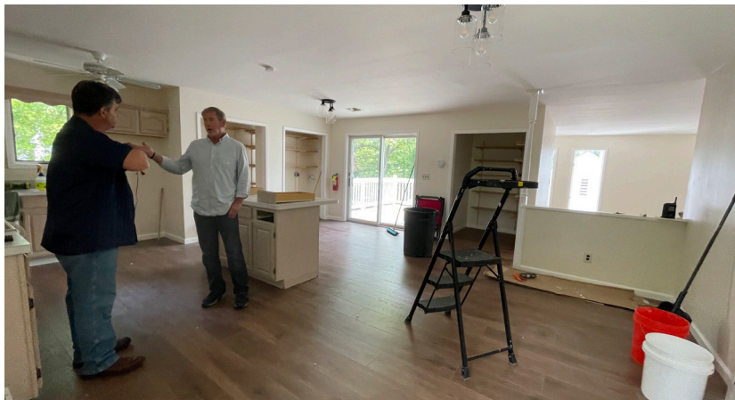
Construction work in process at one of the apartments
